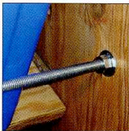
THREADED STEEL rods hold the plywood sides together
